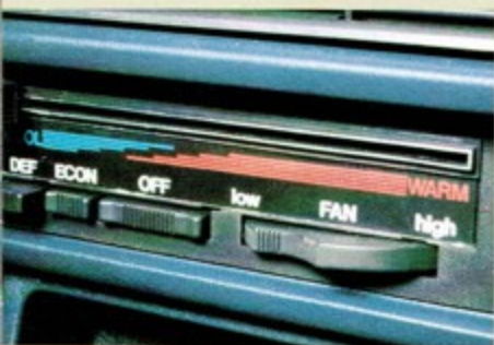
Air conditioning controls integrated into heating/ventilation controls.
